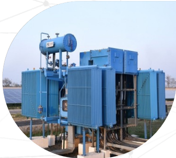
8.8 MVA 33/0.69X2 KV AT 40 MW SOLAR PROJECT AT AYODHYA RAM MANDIR
