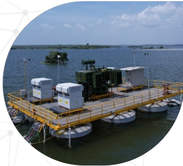
FLOATING SOLAR POWER PLANT: 90 MW 6.6 MVA, 33/0.660*2 KV KNAN IDT at OMKARESHWAR, MADHYA PRADESH
