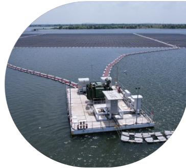
FLOATING SOLAR POWER PLANT: 90 MW 6.6 MVA, 33/0.660*2 KV KNAN IDT at OMKARESHWAR, MADHYA PRADESH
