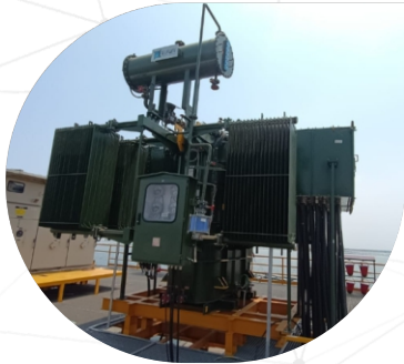
FLOATING SOLAR POWER PLANT: 90 MW 6.6 MVA, 33/0.660*2 KV KNAN IDT at OMKARESHWAR, MADHYA PRADESH
