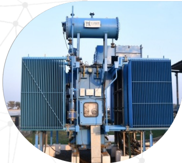
8.8 MVA 33/0.69X2 KV AT 40 MW SOLAR PROJECT AT AYODHYA RAM MANDIR
